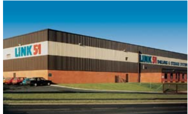
The Shelving & Storage factory at Brierley Hill - once the site of the founding Handy Angle Company
